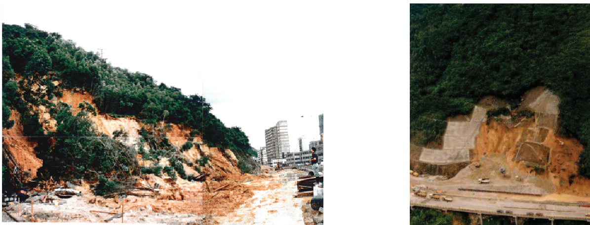
Figure 4: Images of the July/August 1997 landslide within the Ching Cheung Road Study Area (Halcrow, 1998)
